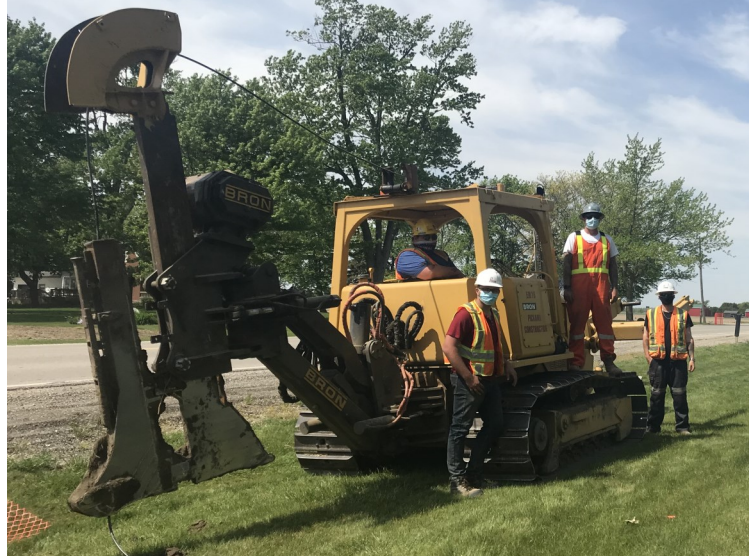
Pickards Fibre Plow Crew on Confederation Line
