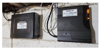
In the basement where the ONT and battery backup were installed, it fits cleanly on the wall (this is one of the many versions of the set up).
